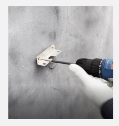
Fix the mounting bracket to the lower screw holes
