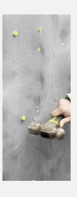
Use the positioning board (included in the charger package) to mark the mounting hole on the wall
